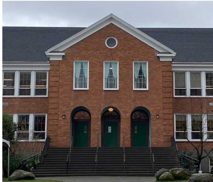
EXISTING - FRONT ENTRANCE (NORTH ELEVATION)
