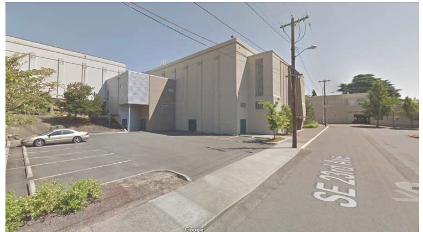
Milwaukie High School, View looking South on SE 23rd Ave
