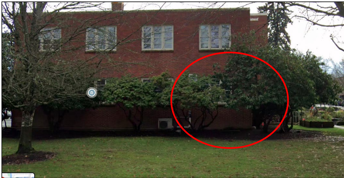
Figure 6. North façade with area of work identified.
