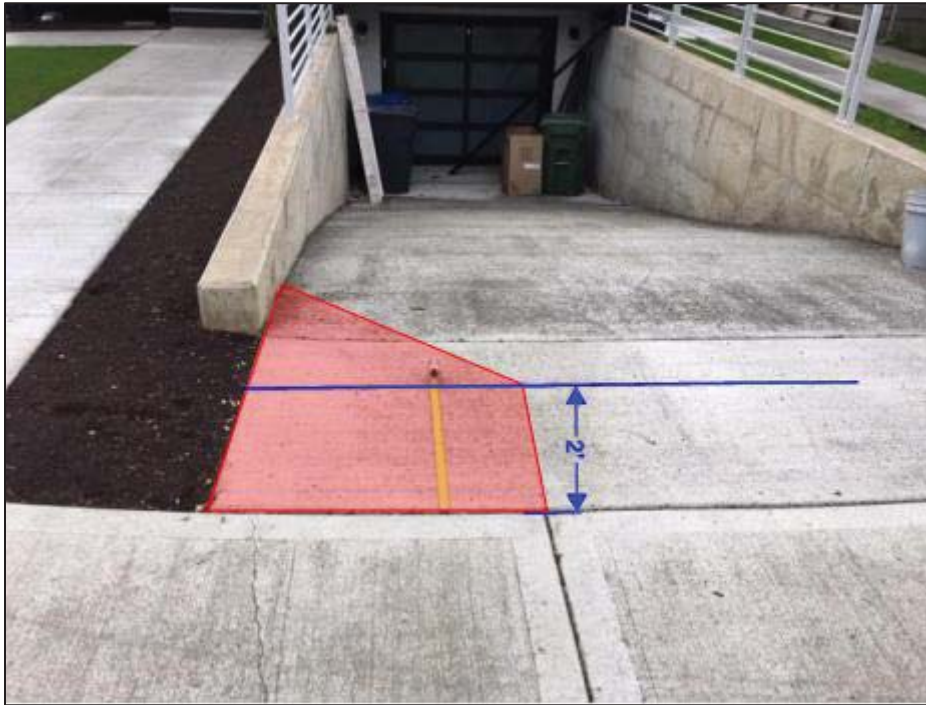
Figure 8. Illustration of driveway area required for removal to comply with MMC 19.607.1.E – Option B
