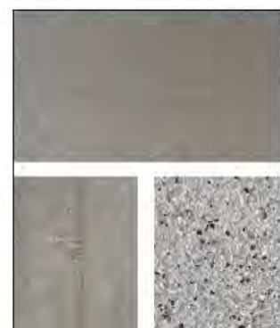
SITE AND PRECAST CONCRETE
