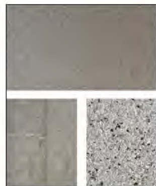
SITE AND PRECAST CONCRETE
