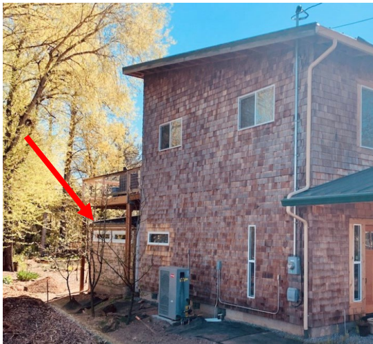
Figure 3. New shed under the deck.
