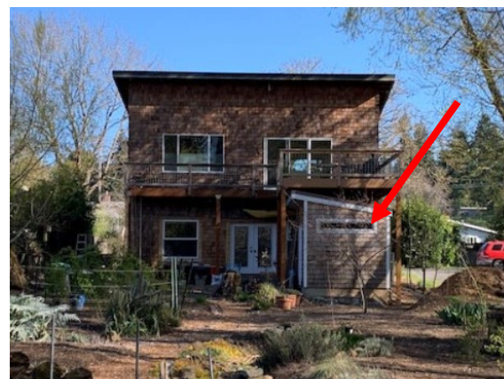
Figure 4. New shed under the deck.
