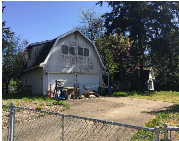
Figure 3. A neighbor's accessory structure to the North.
