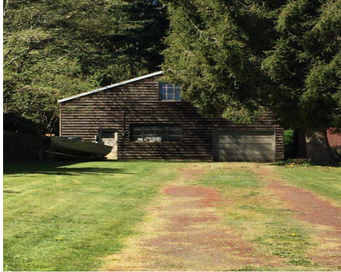
Figure 4. An accessory structure within a few houses of the applicant's.
