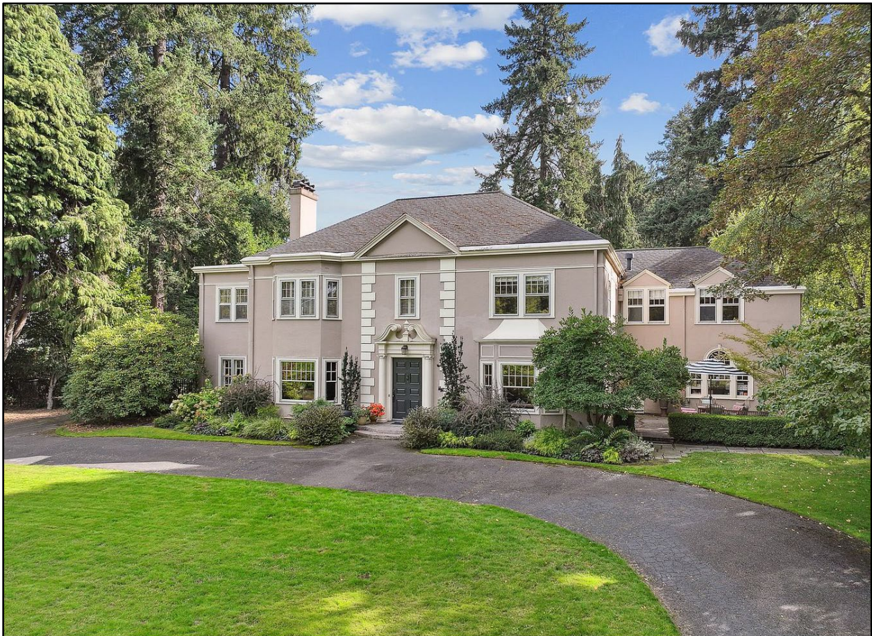
Figure 2.Primary (north) elevation (Zillow)
