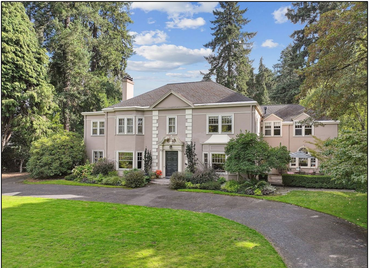
Figure 2.Primary (north) elevation (Zillow)
