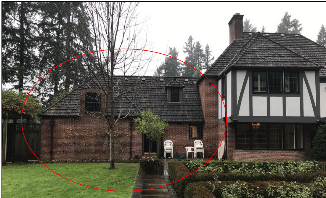
Figure 10. Existing south façade (rear) and location of proposed addition
