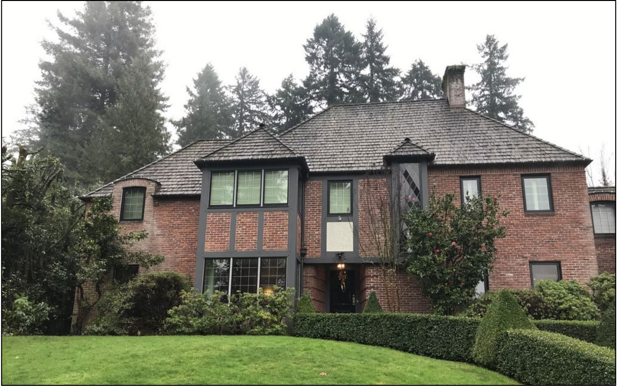
Figure 7. Existing North (street facing) façade – main block of the house
