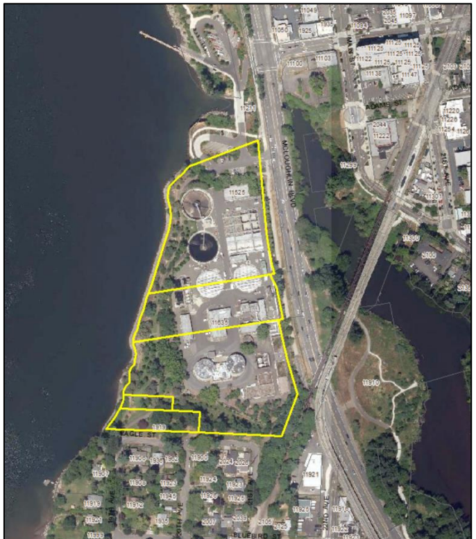
Figure 1. Aerial Photo (subject property outlined in yellow)
