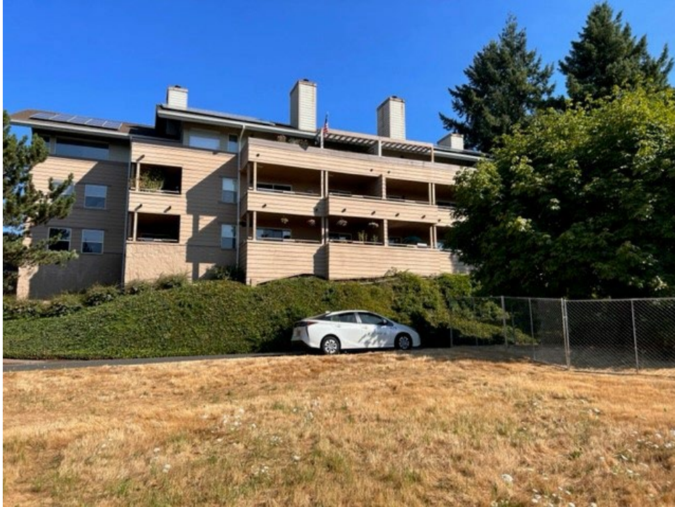
Figure 7. View from site north to Waverly Greens
