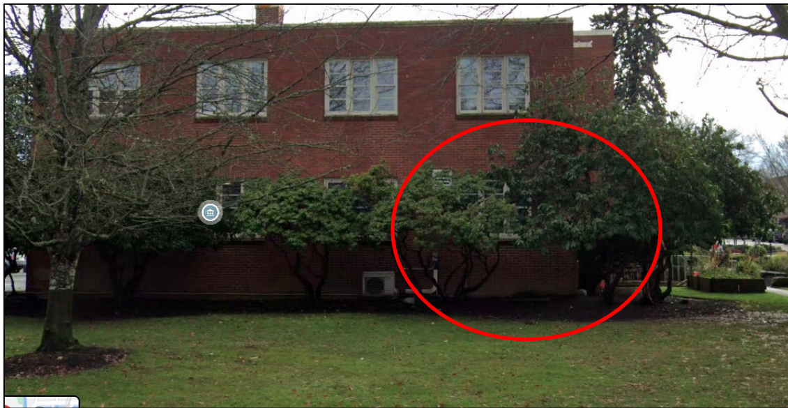
Figure 6. North façade with area of work identified.
