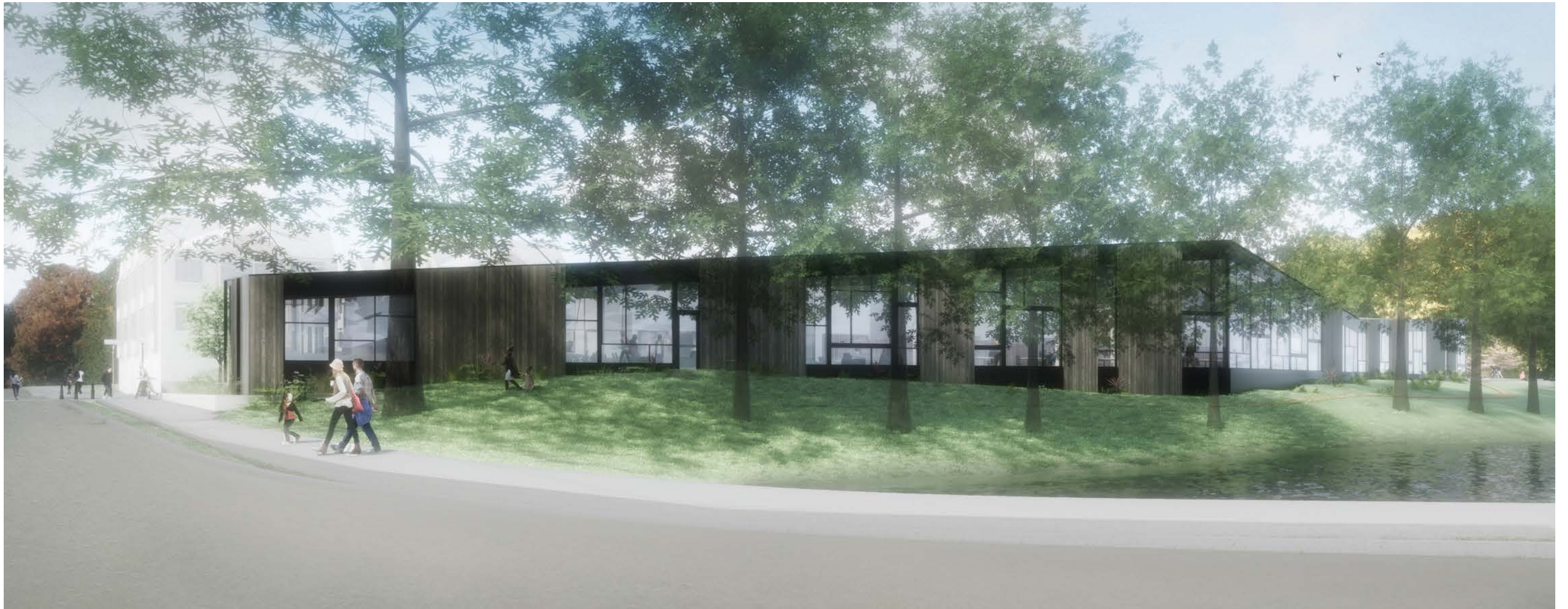
VIEW OF EAST FACADE FROM HARRISON
