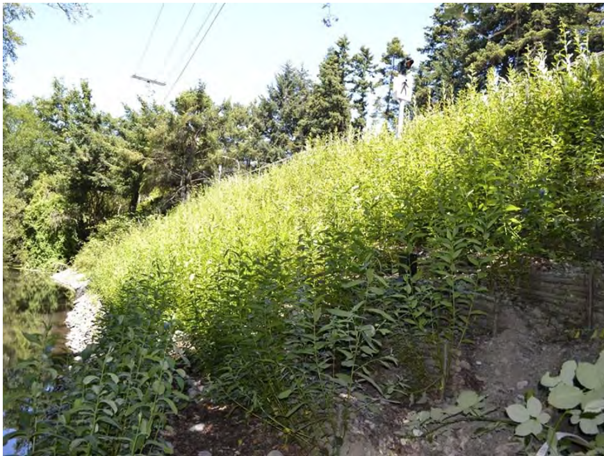
Photo 5. Willow crib wall one year after installation. The willows have sprouted and are forming a dense vegetated slope.
