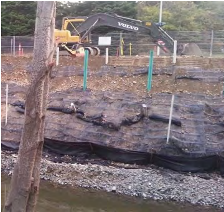
Photo 2. Example of slumping that can occur when a steep unstable slope erodes behind the coir blanket intended to stabilize the slope.
