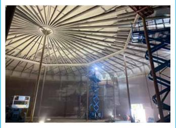
Maintenance work continues on the Stanley Reservoir. Repairs to the tank interior are complete, and crews have begun removing the existing interior coatings and repainting the interior of the reservoir. It's expected that this phase of the project will continue through February 2025. For more information, visit www.milwaukieoregon.gov/engineering/stanley-reservoir-improvement-project.
