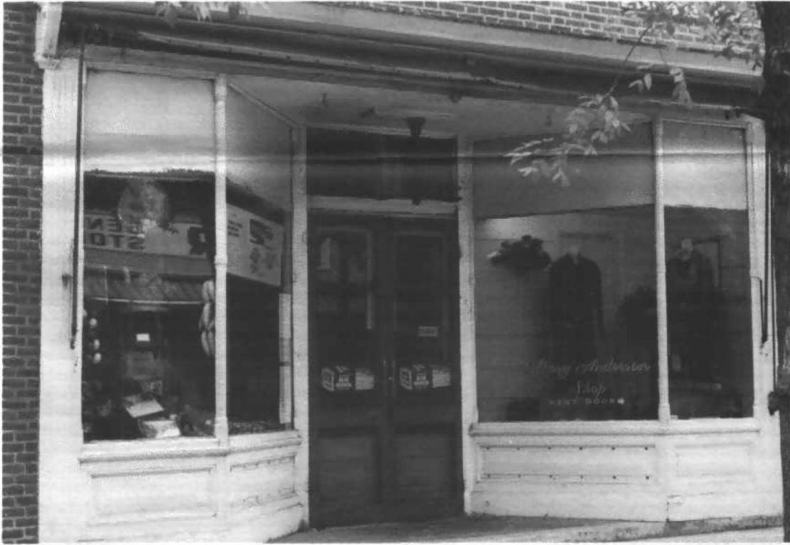
Although Winchester, Va., lost most of its traditional retail anchors to a nearby regional mall, the downtown is attracting upscale specialty shops such as this clothing store.
