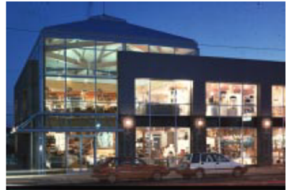
Recommended: Transparency of facade fosters interaction between the public and private realm (NE Broadway and 15th, Portland)
