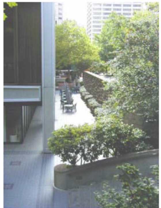
Not Recommended: Seating areas that are depressed or raised from street grade (SW 6th and Main, Portland)
