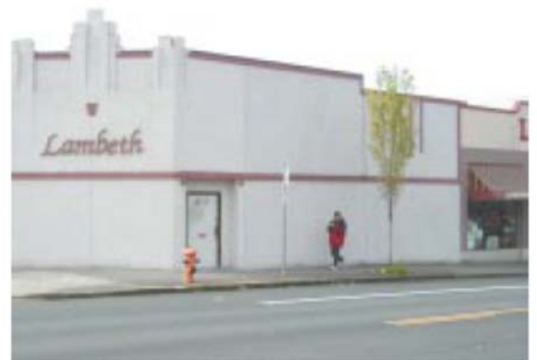
Not Recommended: "Dead edge" created by providing no window openings or building articulation along the lower 15' of the building (N Denver and Schofield, Portland)
