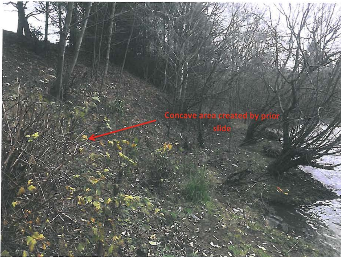
Photograph 4 - From center of bank looking east . The break in slope at the slope toe and concave area above are indicators of a previous landslide.
