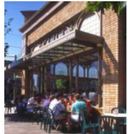
Recommended: Glass and metal canopies integrated into building facade (NE Broadway and 15th, Portland)
