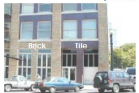
Not Recommended: Facade of historic building is marred by addition of a brightly colored contemporary tile cladding (SW Salmon and 11th, Portland)
