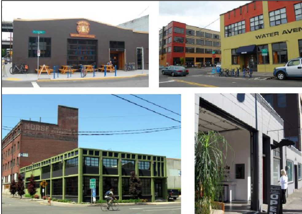
Figure 6. Industrial building retrofits - Portland
