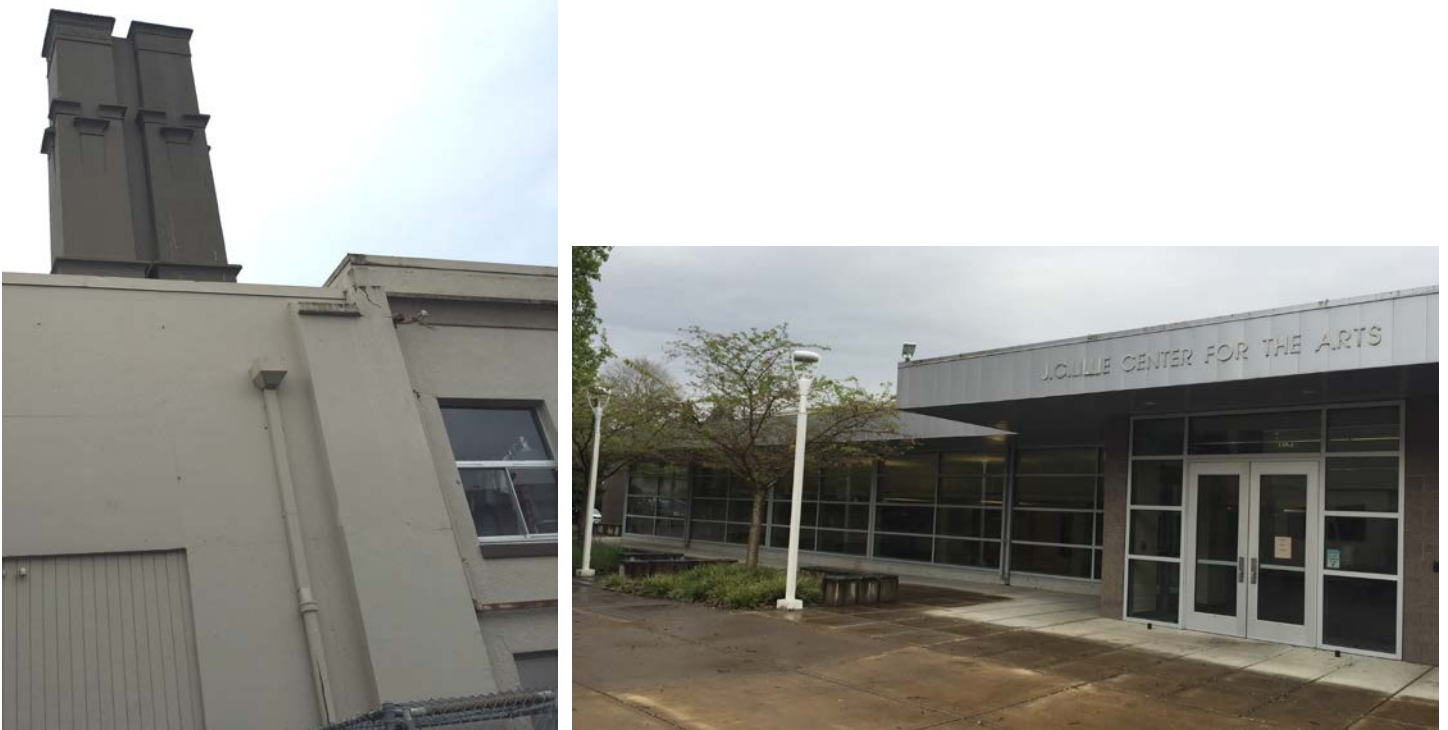
View 10: At left: looking up at the south side of the paired chimneys at the Arts & Crafts/ boiler building. At right: The eastern façade of the J.C. Lillie Auditorium.
