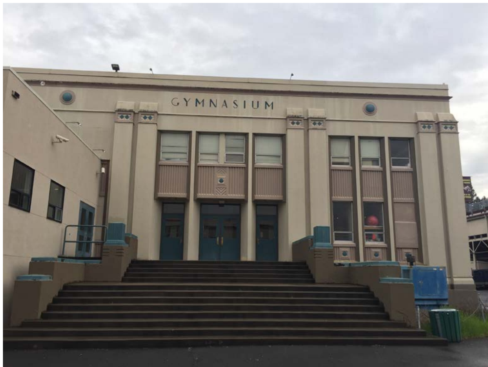
View 9: A portion of the southern façade of the gymnasium, the oldest section of this building.
