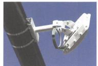
Example of a radar sensor mounted on a traffic signal pole similar to what ODOT will install on existing traffic signals on OR 224/212.
