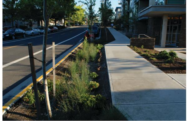
Figure 6. Examples of linear stormwater swales, as proposed for Local Streets
