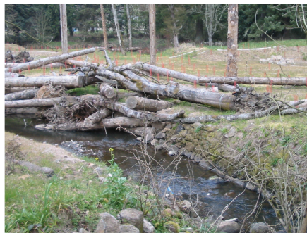
B. Engineered log jams will provide shelter for migrating fish.
