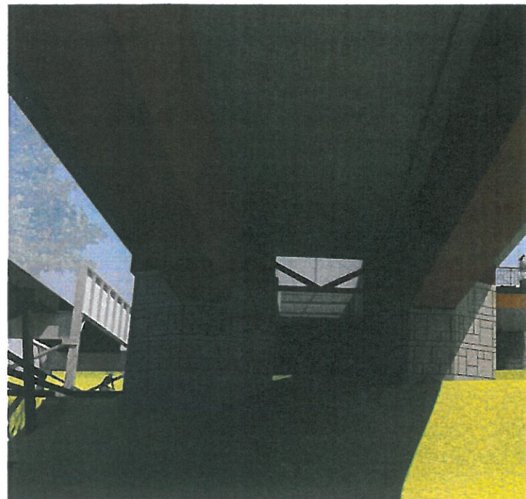
1. View from under Kellogg Bridge in Kronberg Park looking North - Concrete jump span with steel fascia
