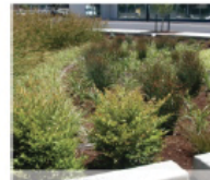
Typical Stormwater Planter
