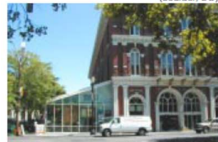
Not Recommended: Addition does not relate well in form, massing or materials (SW 2nd and Ankeny, Portland)
