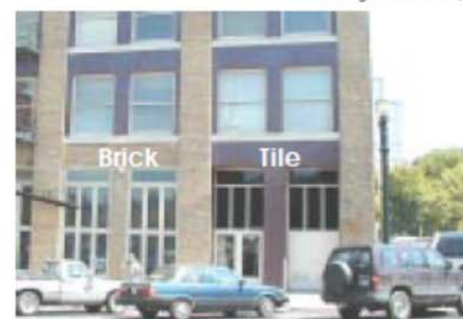
Not Recommended: Facade of historic building is marred by addition of a brightly colored contemporary tile cladding (SW Salmon and 11th, Portland)
