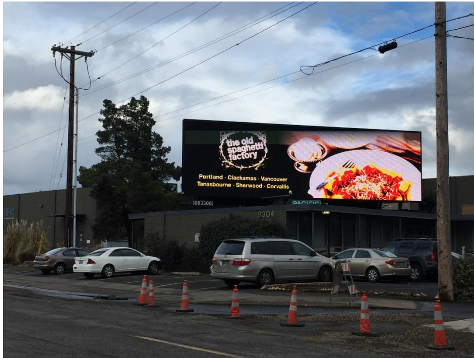
Figure 1. 9304 SE Main St. Area of roof sign is 672 sq ft. Source: Google Earth
