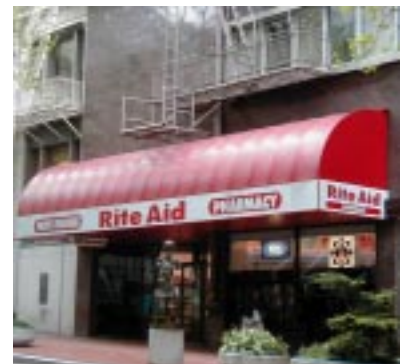
Not Recommended: Vinyl awnings (SW 6th and Alder, Portland)
