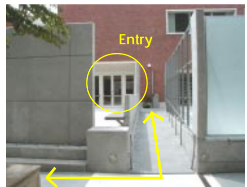
Recommended: Ramp design providing easy access to building entrance without negatively impacting the character of the building (Portland Art Museum)
