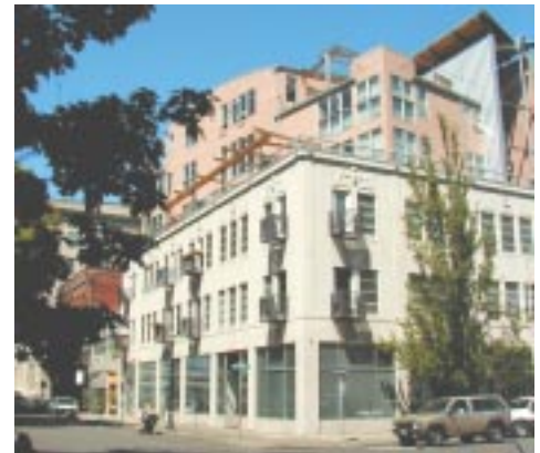
Not Recommended: Contemporary addition on top of historic building contrasts too greatly in form, color and materials with the existing building below. (NW 8th and Flanders, Portland)
