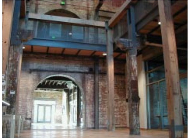
Recommended: Use of salvaged and recycled materials (NW 10th and Irving, Portland)
