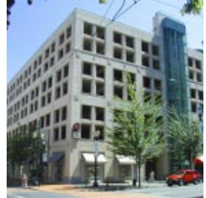
Recommended: Parking garage with ground-floor retail and window-scaled openings (SW Yamhill and 4th, Portland)
