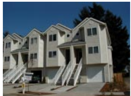
Not Recommended: Entry doors too high above street level (East Burnside and 104th, Portland)
