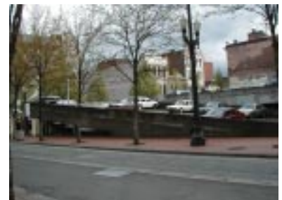
Not Recommended: Exposed sloped parking structure (SW Morrison and 1st, Portland)
