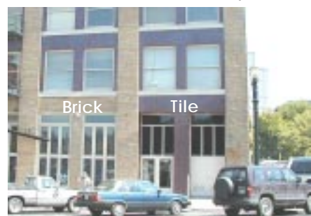
Not Recommended: Facade of historic building is marred by addition of a brightly colored contemporary tile cladding (SW Salmon and 11th, Portland)
