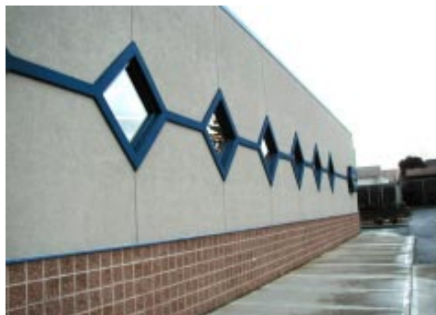
Not Recommended: Horizontal wall character exaggerated by the lack of wall definition and the oddly sized and shaped windows (N Lombard and N Denver, Portland)
