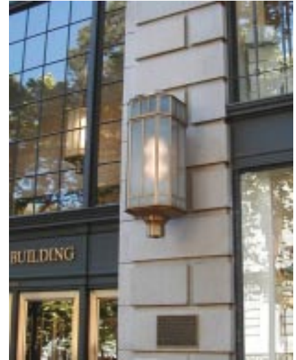
Recommended: Decorative wall sconce designed as part of overall building facade composition (SW Yamhill and 5th, Portland)
