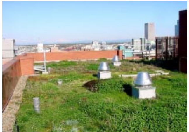
Recommended: Roof that includes landscaping to filter rainwater (SW 12th and Clay, Portland)
