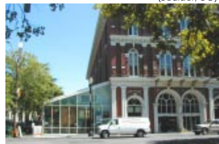
Not Recommended: Addition does not relate well in form, massing or materials (SW 2nd and Ankeny, Portland)
