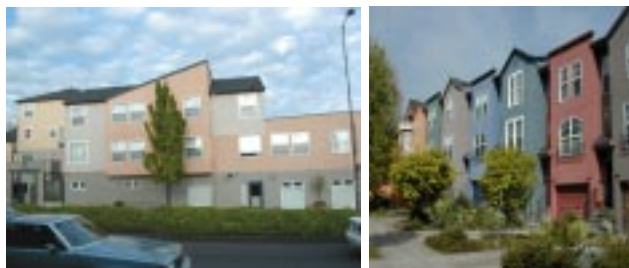
Not Recommended: Walls appear “thin,” lack sense of permanence or have a stage set appearance due to awkward proportions, lack of articulation, use of non-durable materials and bright wall colors (SW Alder and 15th, NW 18th and Lovejoy, NE Skidmore and MLK Blvd., and NW Pettygrove and 23rd, Portland)
