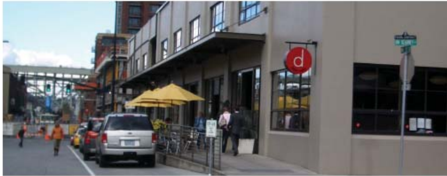
Figure Xc. Retrofitted industrial building with horizontal awnings.
