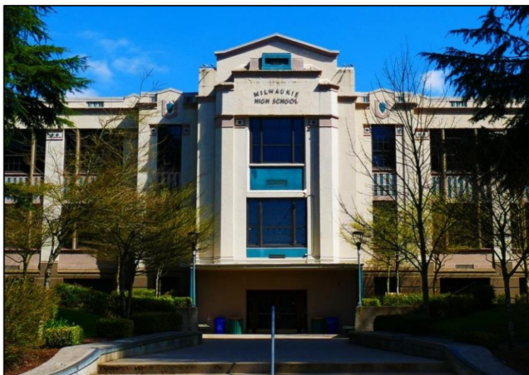
Figure 1. Milwaukie High School (main classroom building)
