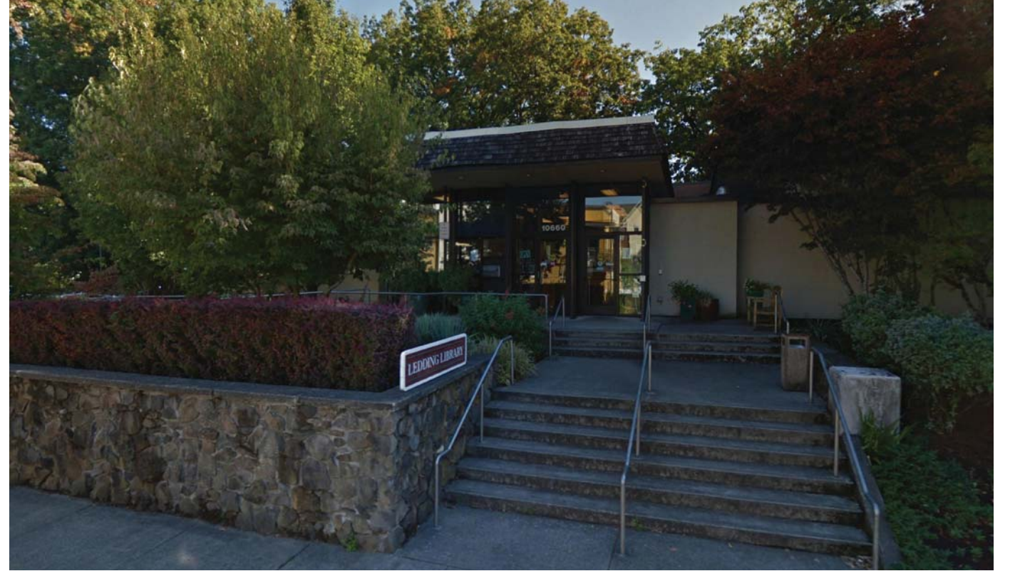
EXISTING STREET VIEW 4 - LOOKING NORTH TOWARD THE EXISTING LEDDING LIBRARY ENTRANCE
