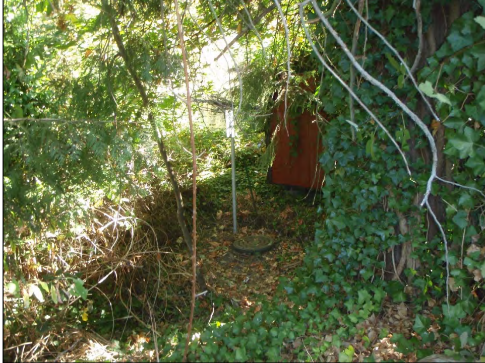
Photo 5. View northwest of manhole. Photo date August 25, 2016.
