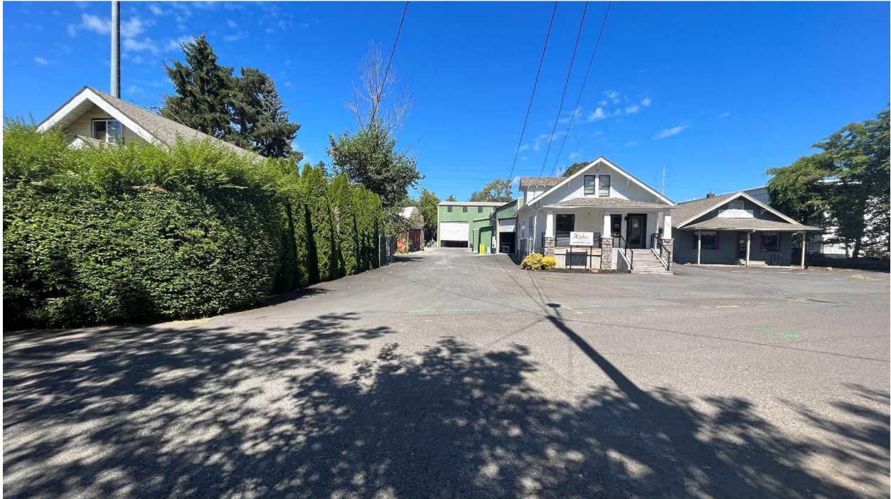
As-Built. The building section facing the street with the 3 window panels and white roll-up door is the building we propose to extend.
