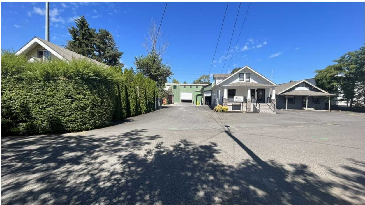
Proposed: note the back warehouse continues to the West, or Left in this rendering.
