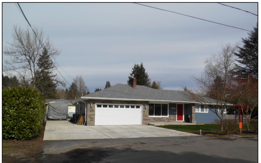
Figure 1. Improved driveway at subject property (Feb. 2019)
