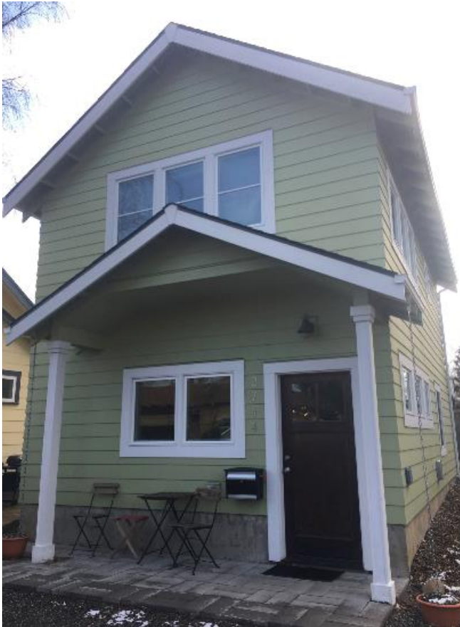
Figure 3: An ADU that has been successfully designed, permitted, constructed, and lived in.
